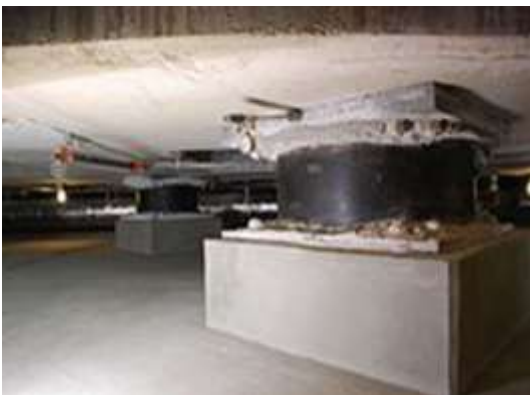
The base isolators under the Utah State Capitol building
